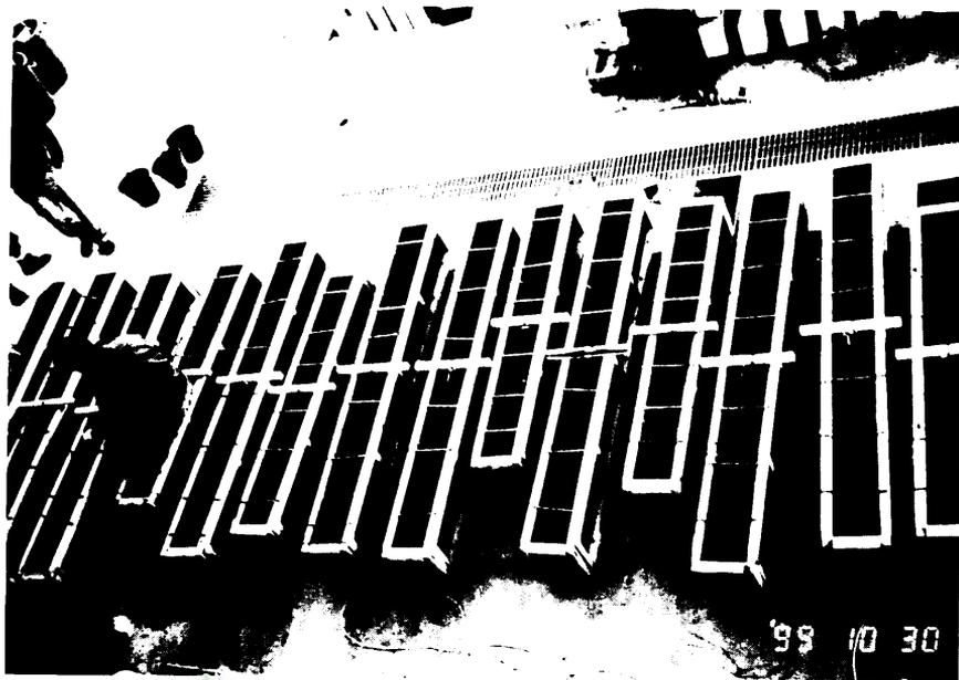
Photo 5 Placing of assembled steels in forms
