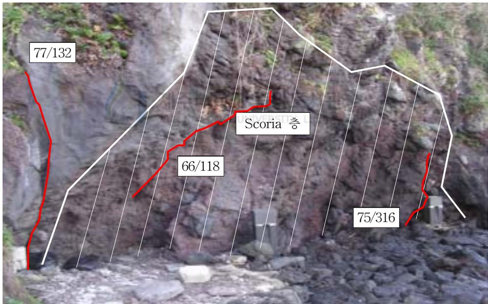
Fig. 4.19 Photograph of scoria layer of the lower part of slope in 2 zone
