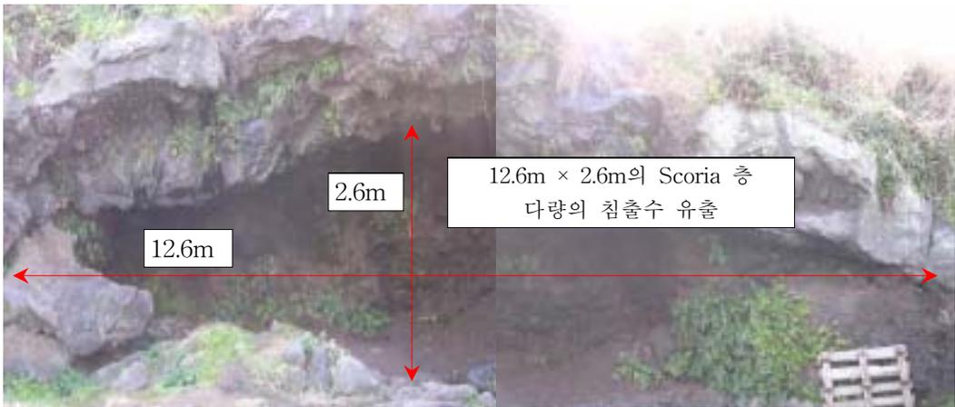
Fig. 4.21 Photograph of cavity by scoria layer weathering
