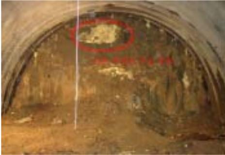
Fig. 3.14 The condition that grouting is completed with Steel pipe urethane
