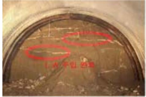
Fig. 3.15 The condition that grouting is completed with L.W
