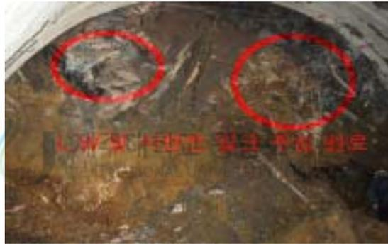
Fig. 3.16 The condition that grouting is completed with L.W, Cement milk
