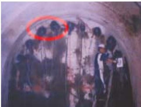
Fig. 3.8 The condition that grouting is completed with steel pipe multi-step grouting, 1
