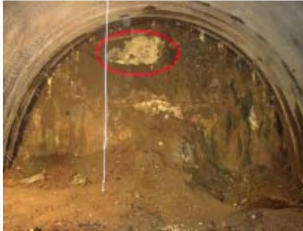
Fig. 2.2 Fracturing grout
