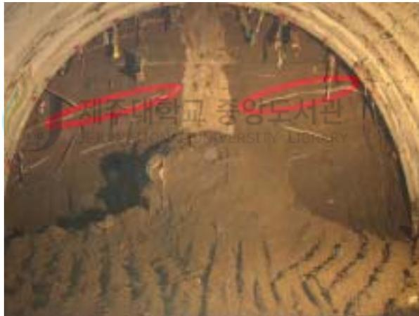
Fig. 2.1 Permeating grout
