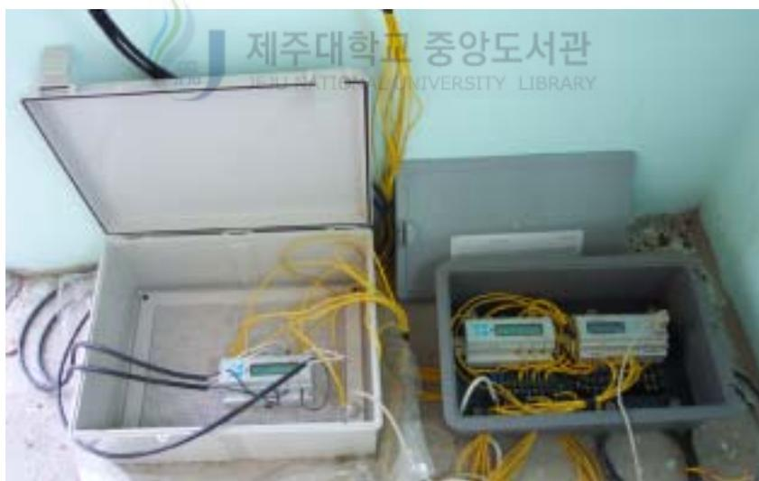
Fig. 3-8 Measurement apparatus for power consumption
