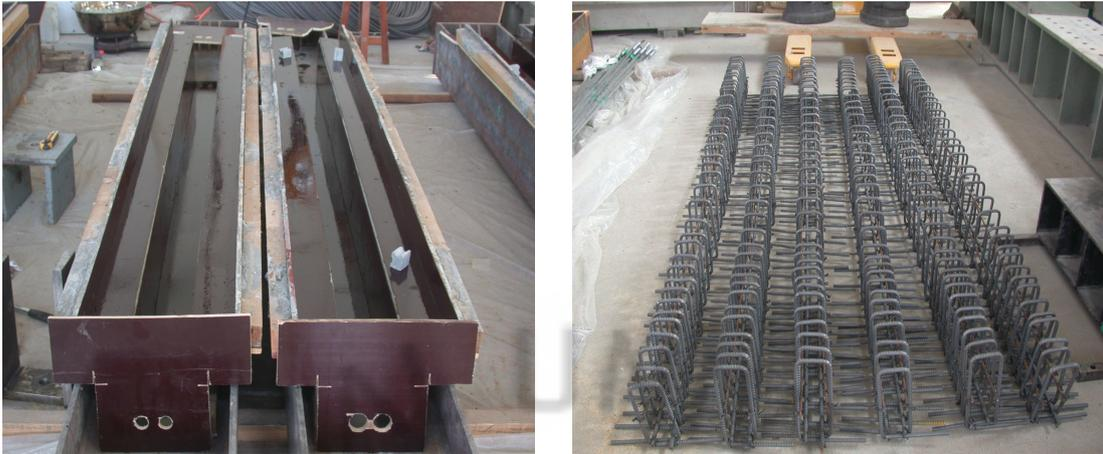
Fig. 3.2 Form and reinforcement arrangement for stirrups
