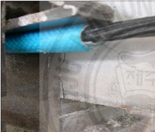
(c) Cracks around deviator
